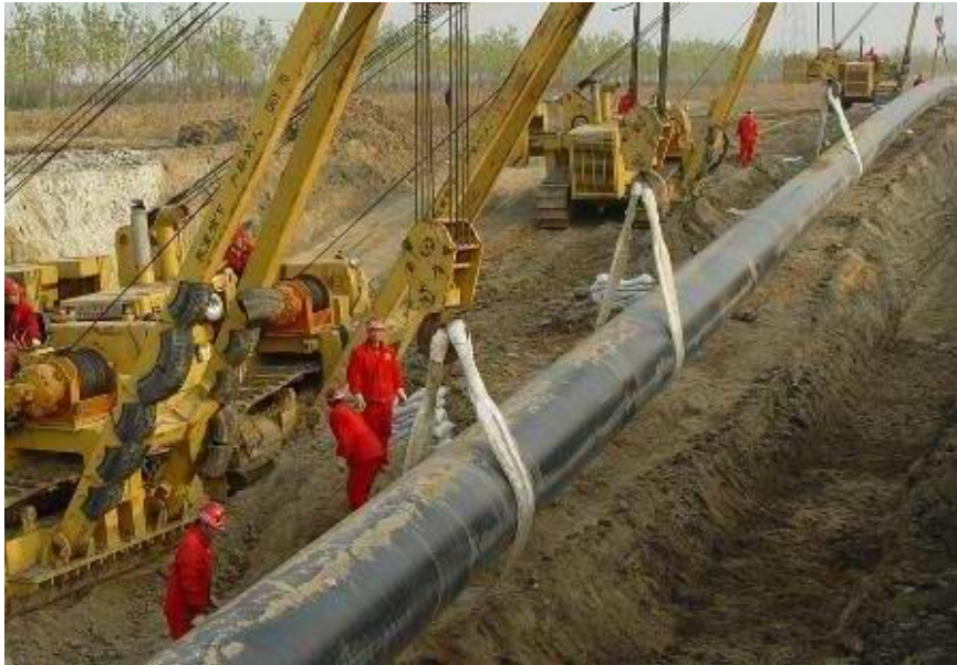
Figure 3-6 Construction of the second natural gas transferring project to Beijing.
